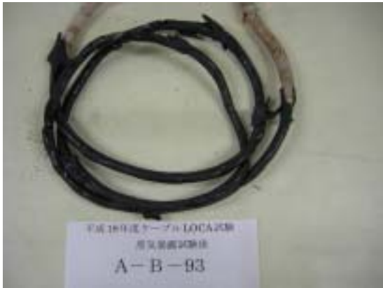
Fig. 2.4.2-20 Specimen A-B-93 after steam exposure test
